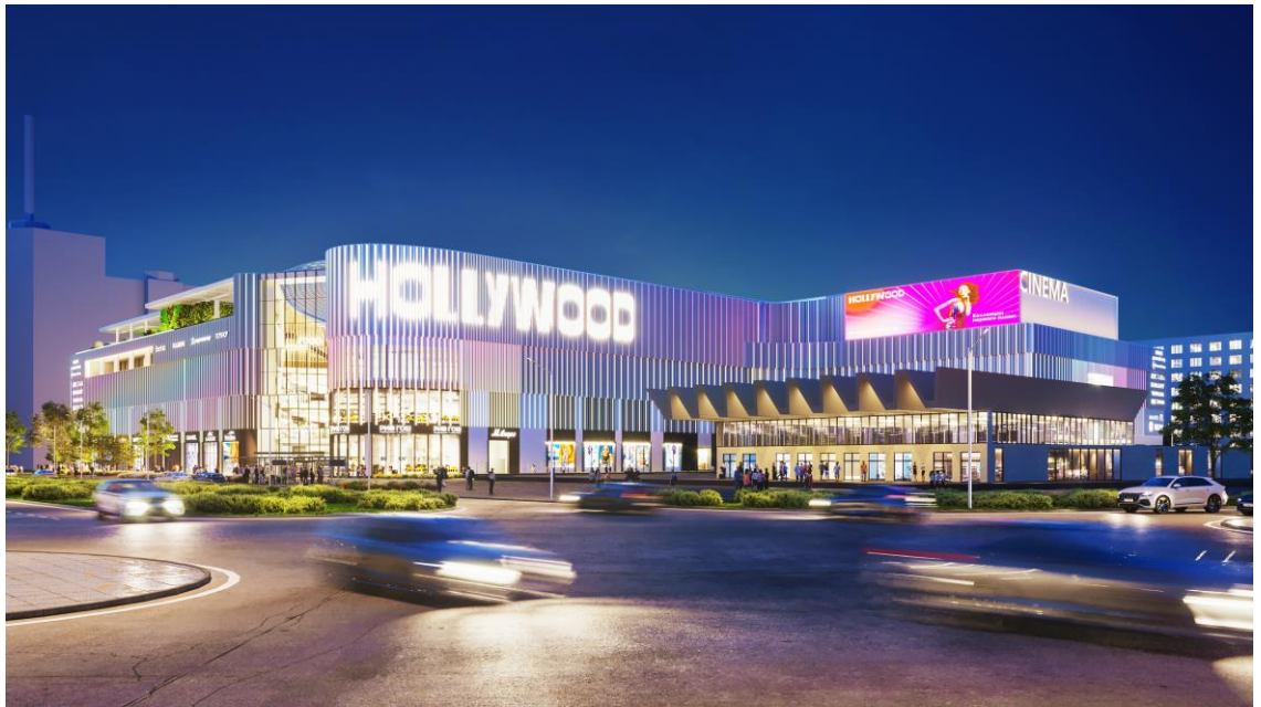
The largest mall under construction in St. Petersburg – MFSEC HOLLYWOOD
